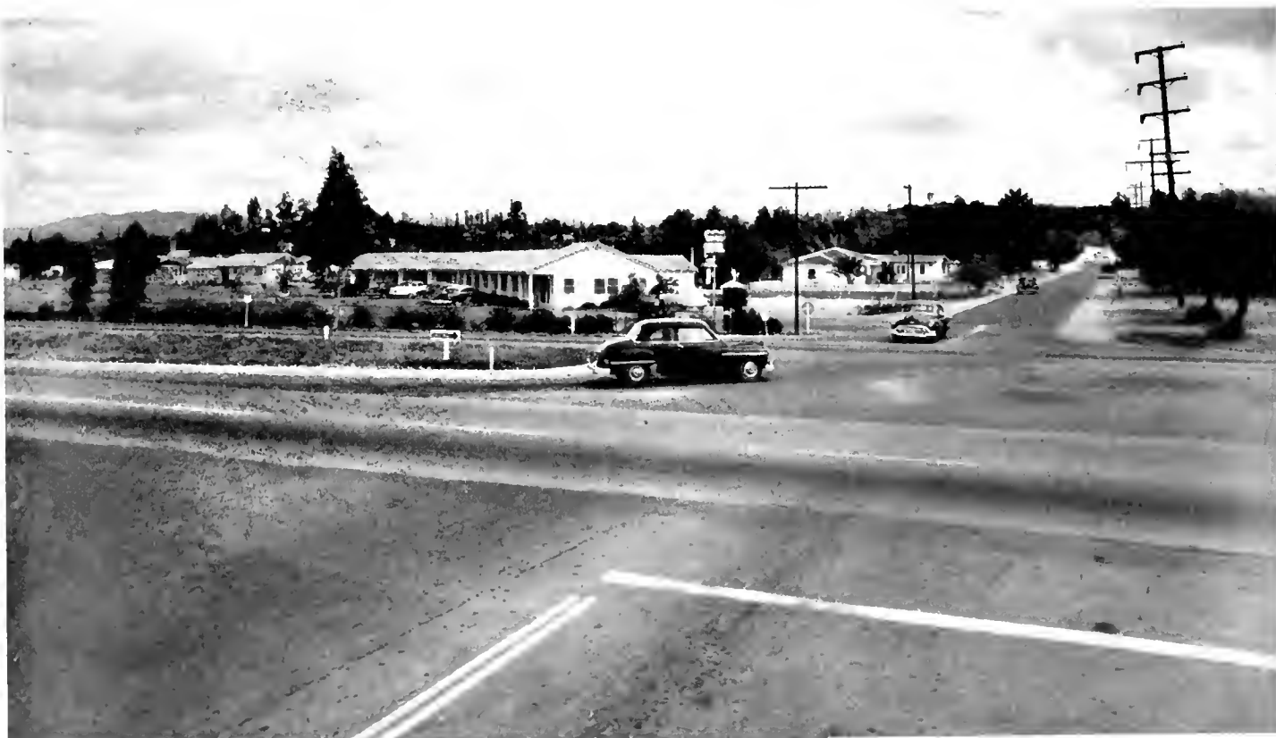
PHOTO 2—Motel along expressway in Escondido. Fence across front of property confines motel entrance to side street. Entrance visible in right center portion of photo beyond expressway intersection.
